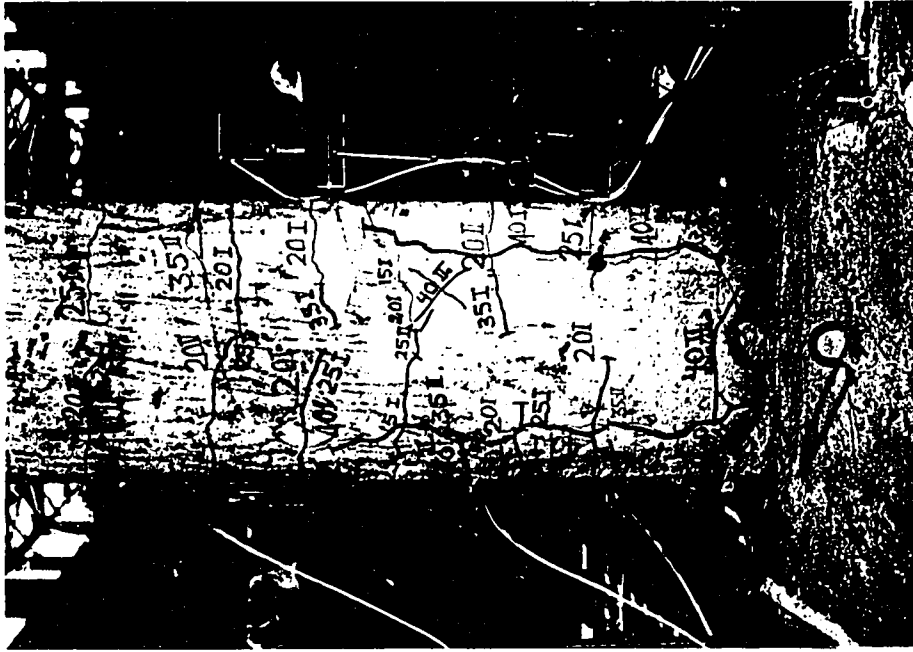
(b) Crack pattern at the splice, south side
