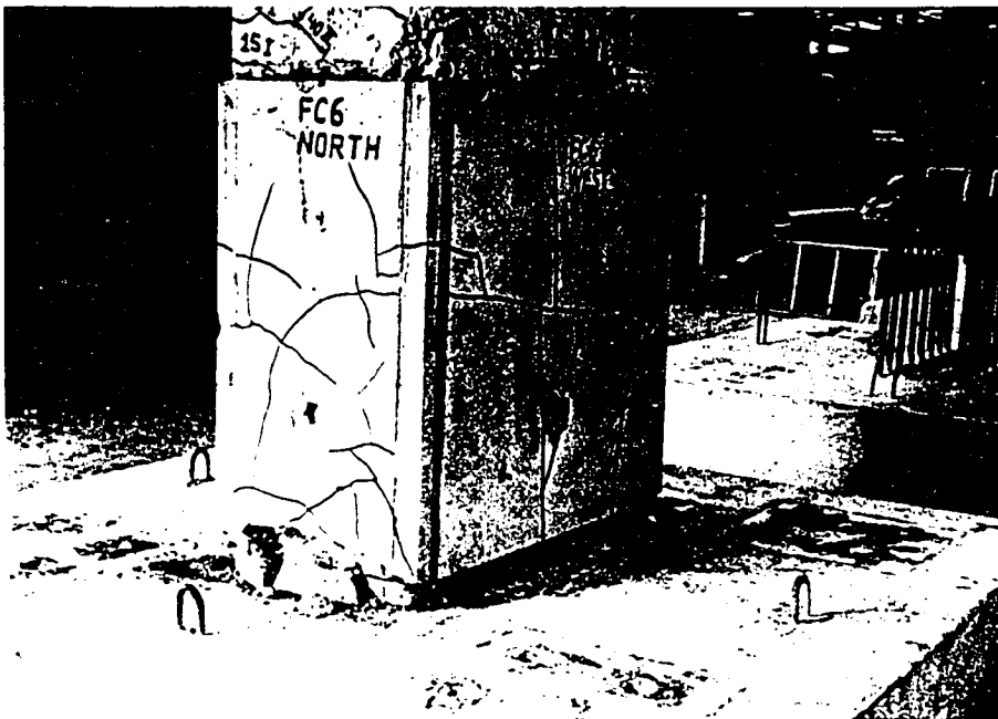
(b) Crack pattern on non-shrink grout, N-W side
