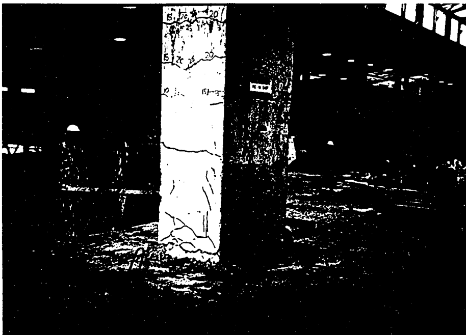
(b) Crack pattern at the splice, S-E side
