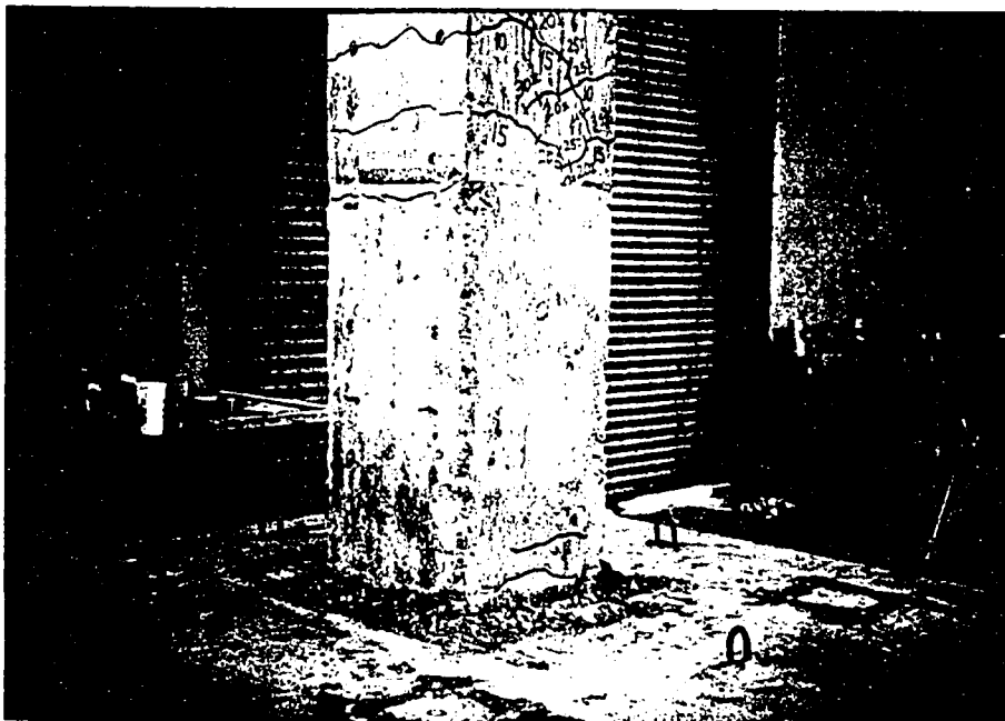
(b) After the removal of the steel jacket, S-W side
