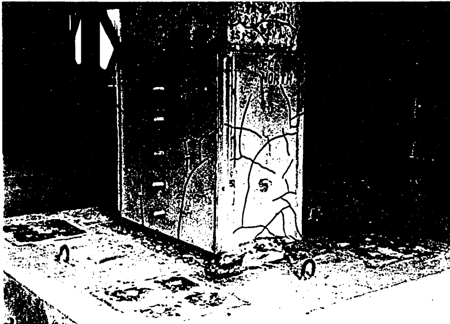
(a) Crack pattern on non-shrink grout, N-E side
