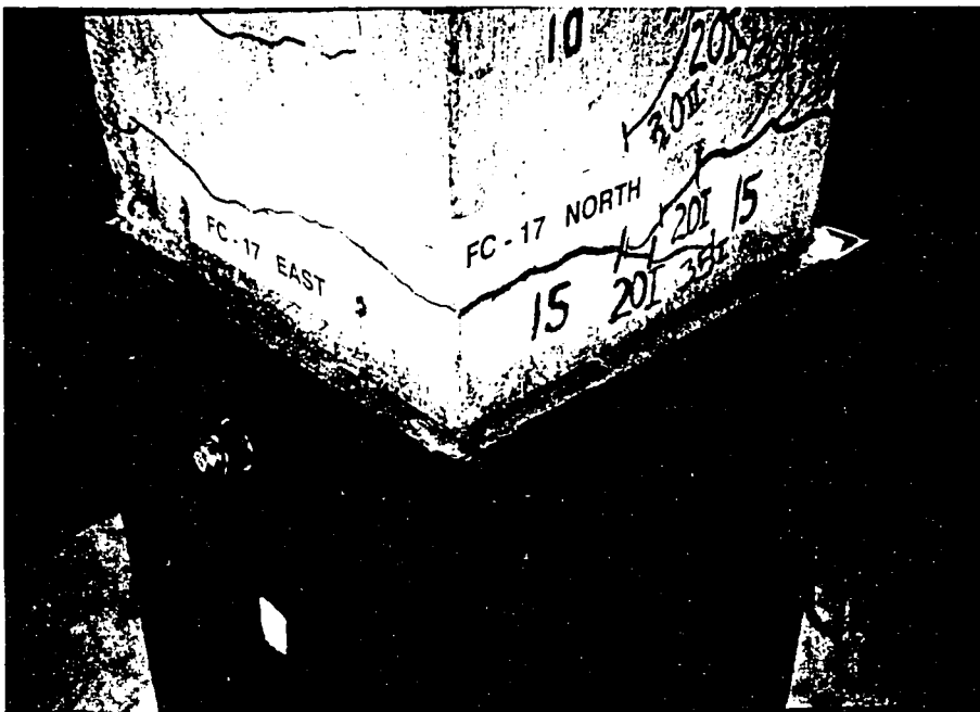
(b) Corner view of the steel jacket
